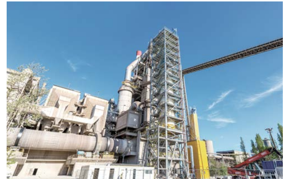
At the HeidelbergCement plant in Lixhe, Belgium, the LEILAC consortium is working on capturing CO 2 in its purest form, thereby reducing the ecological footprint of cement production.
