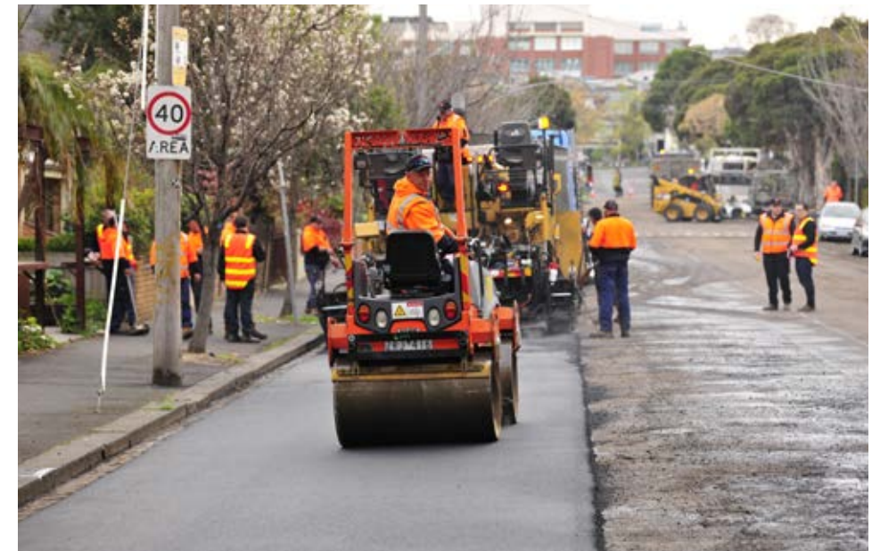
The asphalt mix Green Roads PolyPave from our Australian subsidiary Alex Fraser Group contains recycled plastic and offers numerous environmental benefits.
