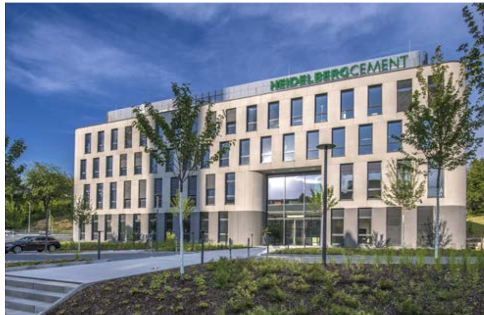
The Heidelberg Technology Center (HTC) in Leimen, Germany: one of the main focuses of research here is the reduction of CO 2 emissions.
